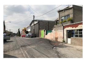
A large crack cuts through this Mexico City street. Half of the street is lower than the other half, one of many signs this metropolis is sinking.
